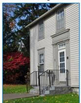
the transom; a modern door has been installed; the foundation has been stuccoed and the front cellar window stoned-in; cement steps have been installed and a pediment replaces the original entabla-
